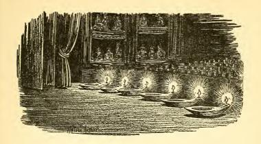
THE first attempt to use footlights for stage illumination is credited to Nicola Sabbatini, an Italian producer, working in the early part of the seventeenth century. About 1620 he designed a parapet to be erected at the front of the stage with a row of oil lamps placed behind it. So This rudimentary and meagre arrangement was the first step in the development of footlights in the modern theatre.
